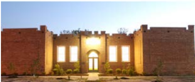
Old Waveland Elementary School post-Hurricane Katrina in 2005, and after restoration in 2008. Image credit: unabridged Architecture
