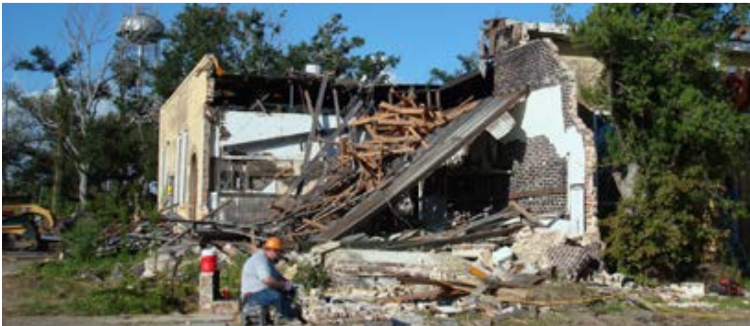
Brick salvage | Image credit: unabridged Architecture
