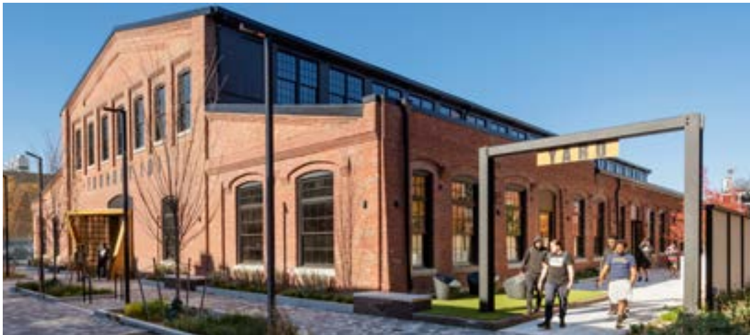
Foundry IO1, Exterior Post-renovation | Image credit: Anton Grassl courtesy of CambridgeSeven
